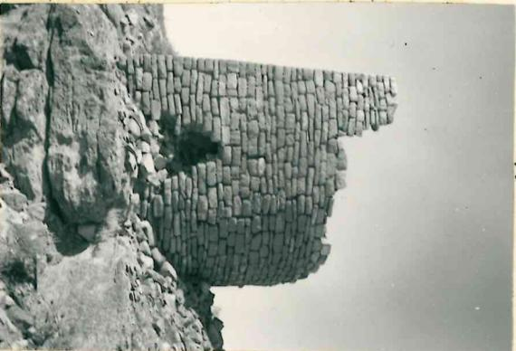
A and B are different views of the same building; in A, above, is shown a small hole at its base which should be repaired (holes such as this one expand rapidly throughout the years, unless repaired, and ultimately the structure is reduced to an uninteresting pile of rocks, of little instructive value to the ordinary visitor); in B, below, lack of bonding, and
