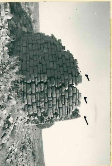
weathering has split the semi-circular wall into three wobbly divisions, indicated by small check marks.
