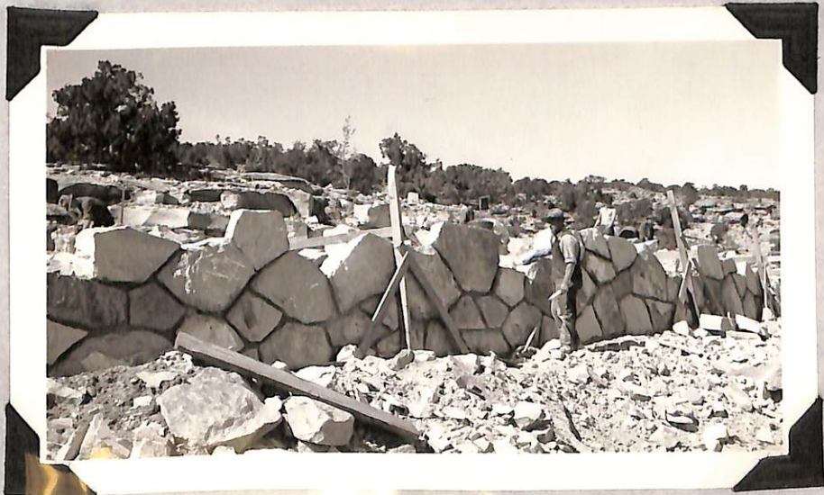
Rubble masonry wall Station 444 Section A
