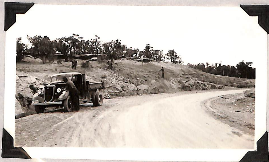
Two views of bank sloping in Section D.
