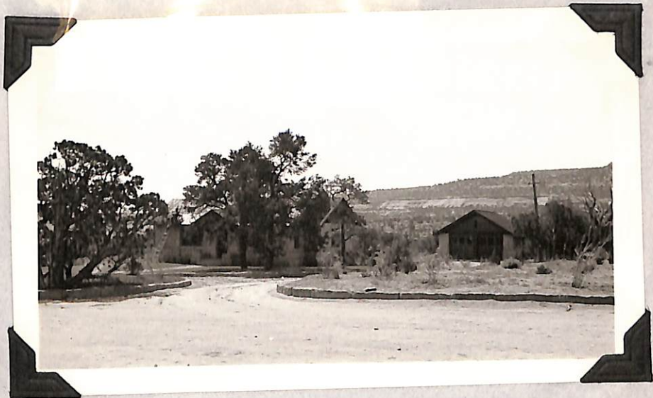
View of completed garage
