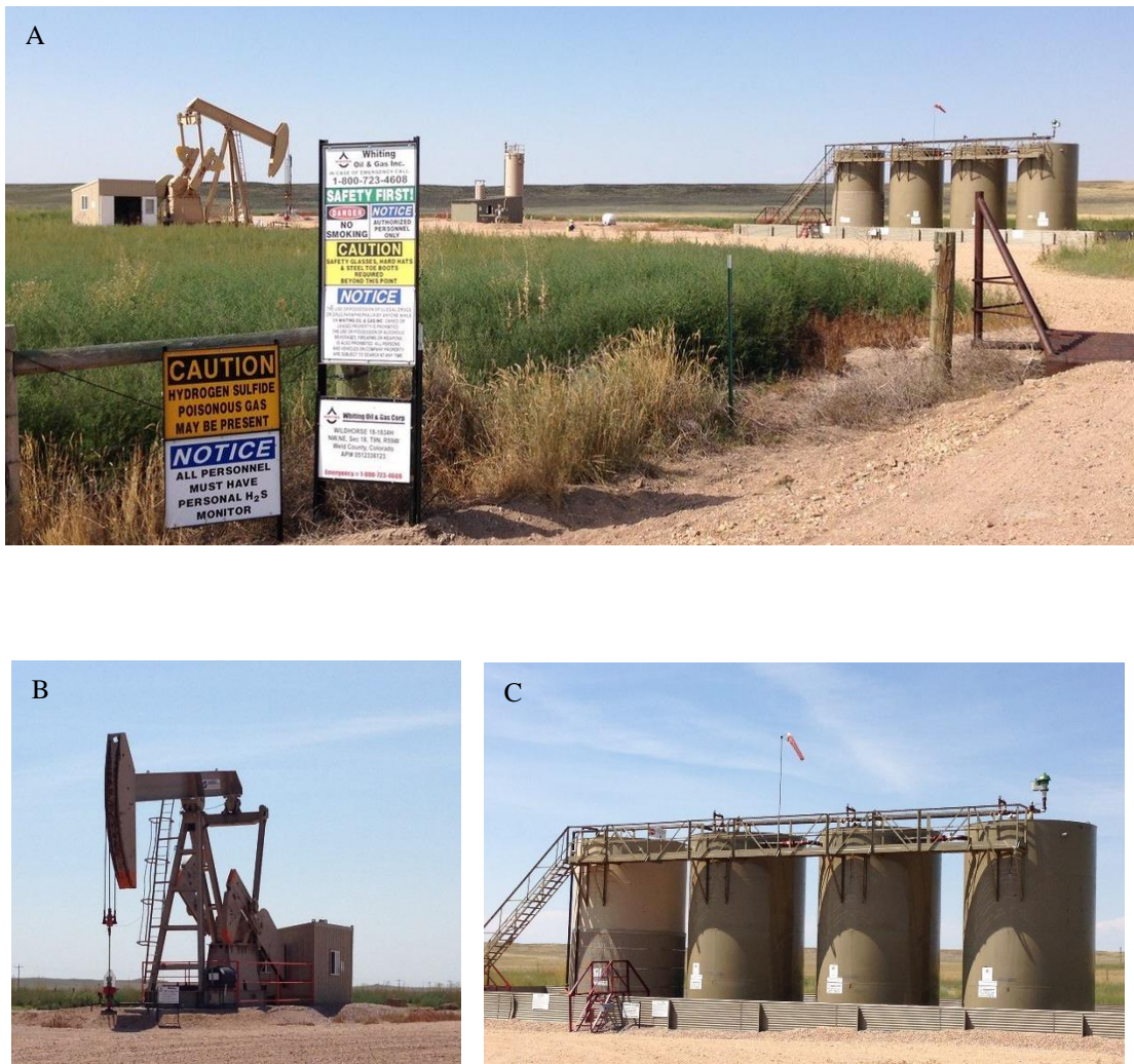
Figure 2. Example oil and natural gas site infrastructure on the Pawnee National Grassland. A = Full site, B = pumpjack, C = condensate tanks, D = Evaporation pit, E = older tank and stack.
